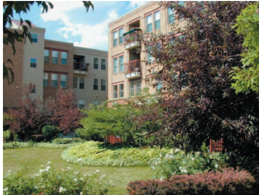
River Station (Minneapolis)
